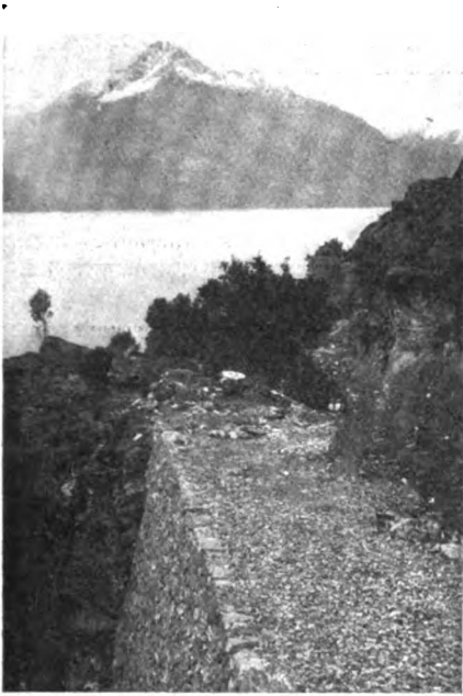
Lake Wakatipu and Road Embankment.
